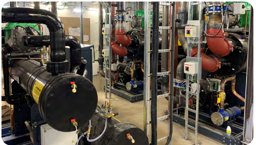
Ringsted installation of Geoclima heat pumps utilizing Danfoss Turbocor oil-free compressors with Solstice® (R-1234ze) refrigerant. Image courtesy of Danfoss.
